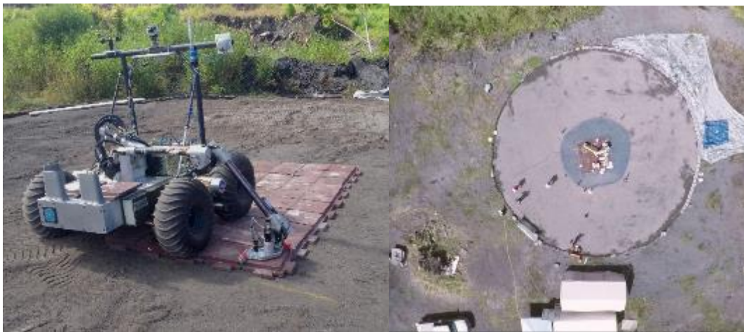
Figure 3: PISCES Rover Helelani (left) using Honeybee Robotics robotic arm during the construction of vertical landing pad using pavers made with Hawaiian basalt, and the completed pad & apron prior to rocket engine test (right).
